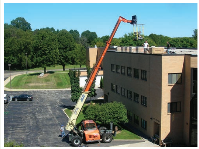
Solar panel installation at Cedar Lake Health and Rehabilitation Center
