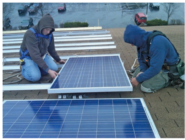
Solar panel installation at Cedar Ridge
